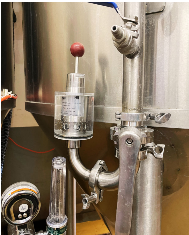
Spunding valve used in the CO2 capture process.
