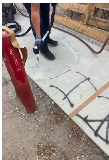
DRY ICE BLASTING TECHNOLOGY USED TO REMOVE GRAFFITI
