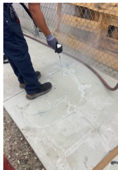
DRY ICE BLASTING TECHNOLOGY USED TO REMOVE GRAFFITI
